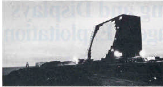
The Cobra Dane phased array radar outpost in the Aleutian Islands, Alaska, will receive new computers and electronics components to improve data collection and processing.
